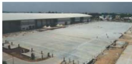
Construction of Hall 5 is in progress. In the first phase, flooring for the hall has been completed and we expect the hall to be ready by July 2018. This hall will be identical to Hall 4 with 75 mts. span and 235 mts. length. With completion of Hall 5 construction, BIEC will have a gross space of around 77,000 sq.mts.
